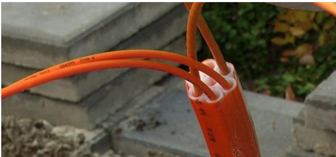
Figure 4. Installation of a multiduct system [15]
