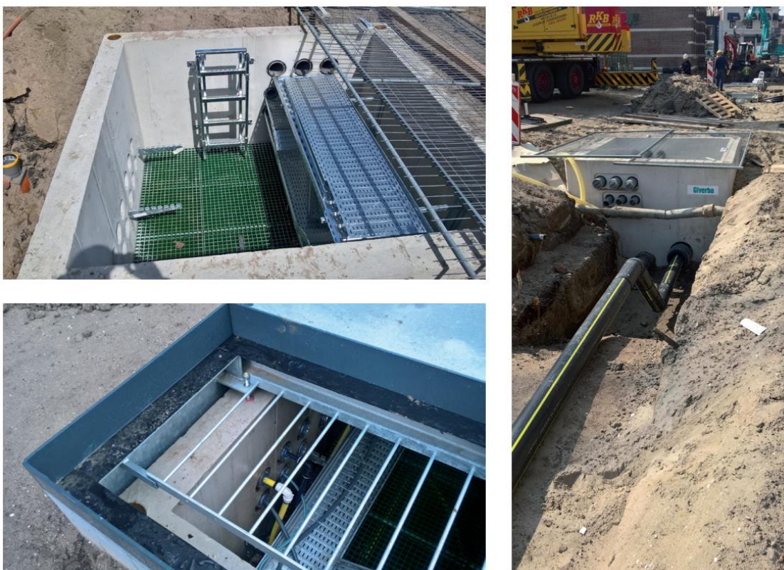
Figure 3. Example of inspection manholes in a shared pipeline route [14]
