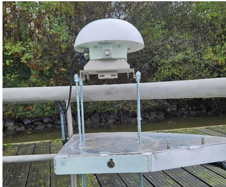
Figure 71 Increased height of communication to provide LoS links.
