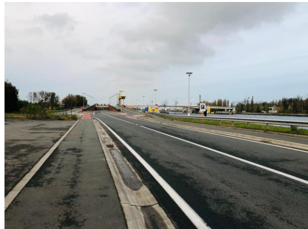
Figure 27 - Picture taken in Zelzate site
